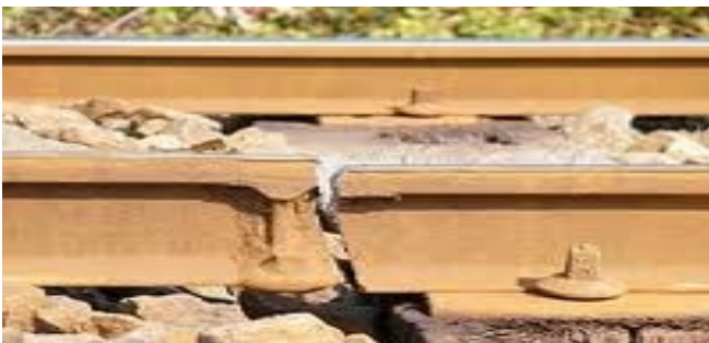
Fig 2. Crack in rails
